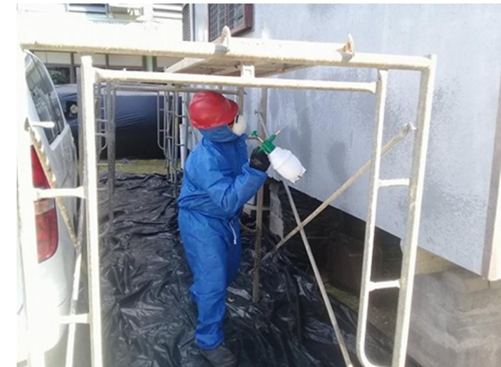
Wet Spray method using base mixture
