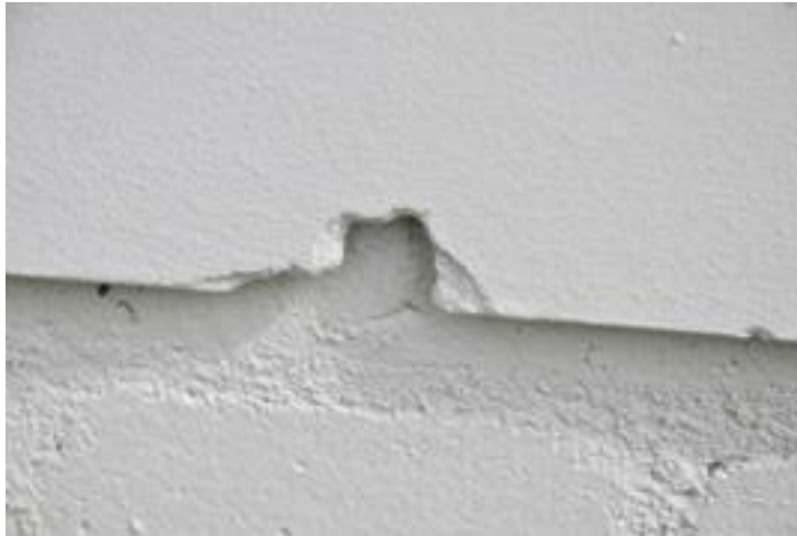
Edges and surface of solid external cladding sealed with paint - non-friable
