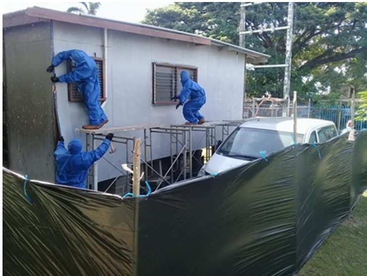
ACM Removal to test building MCILI
