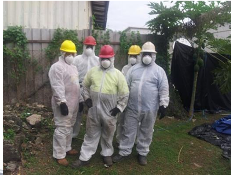
Workers in PPE before works starts on second day
