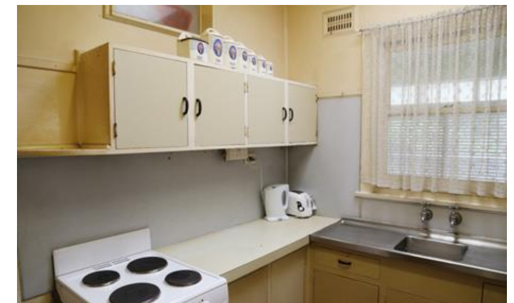
Kitchen cladding and tile splashback
