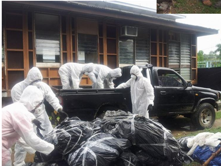
Safe storage on site and disposal to a designated site onto vehicle
