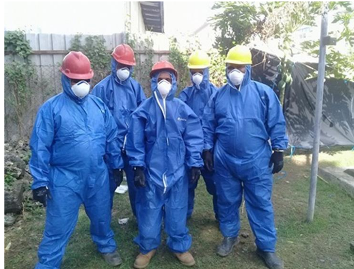
Workers in PPE at the start of the work
