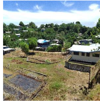
Figure 23 – Foundations from earlier phase works and Naha 1 east side residence
