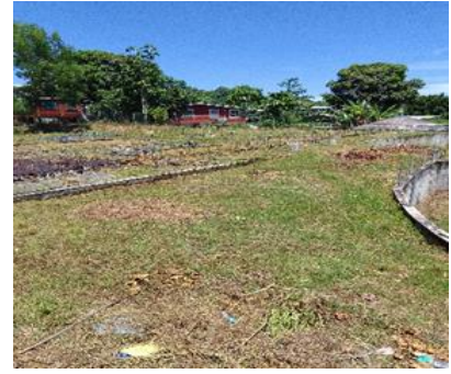
Figure 32 – Earlier phase foundation works looking west from existing clinic
