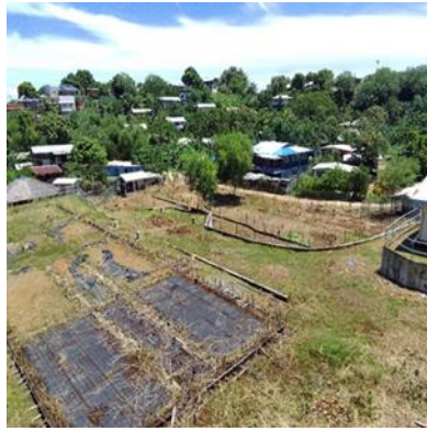
Figure 22 -Foundations from earlier phase, looking east from south hill
