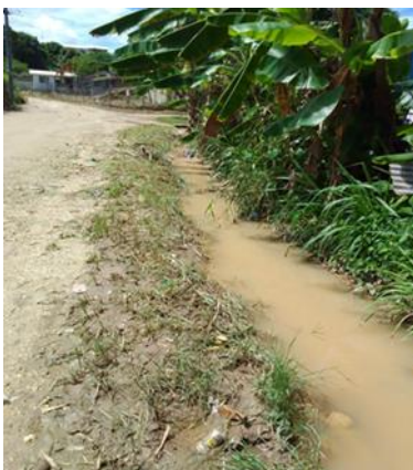
fig Figure 27 – Feeder road going to project site and offside drainage
