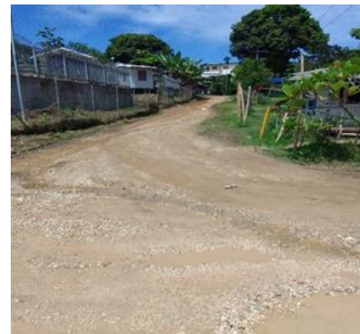
Figure 26 – Feeder road directly next to site on northern boundary
