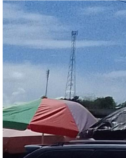
Figure 12. Kombito communication tower
