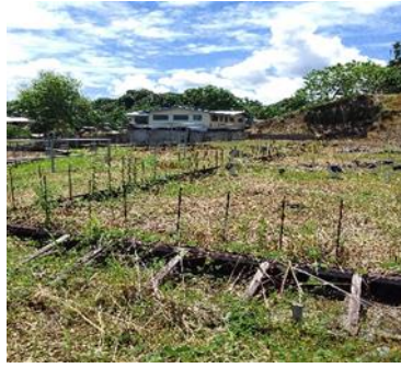
Figure 31 – Foundations from earlier phase looking north from Existing clinic
