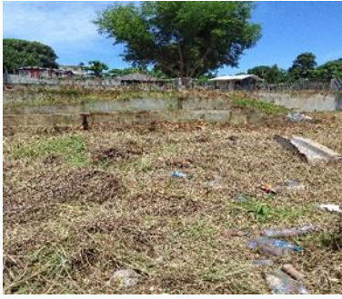
Figure 30 – Foundations works from earlier phase looking from east section
