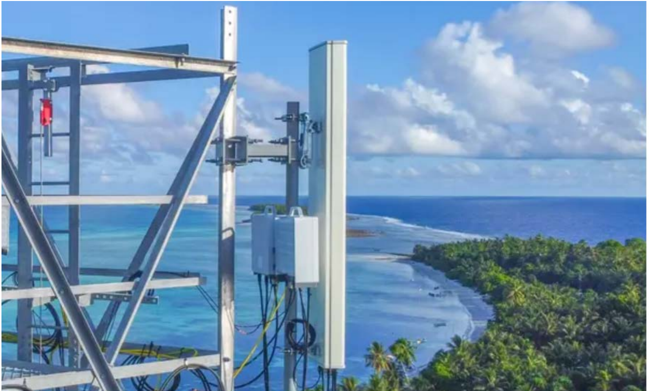
The new tower at Pelau, Malaita Province 1
